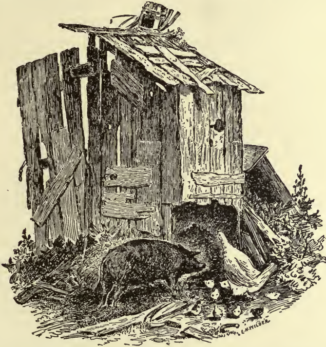
Fig. 92.—An insanitary privy, found too frequently on our farms. Notice how the animals are spreading soil pollution. (Public Health Reports.)
